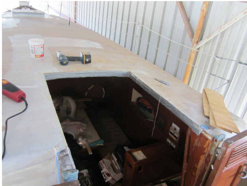
Fiberglass of cabin top in progress
